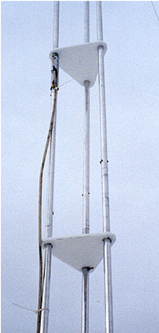
Figure 7—A view of the plastic breadboard insulators and the 40-meter feedpoint 14 feet 9 inches from the base of the 40-meter element.
